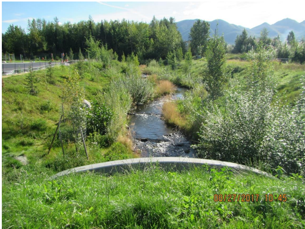
Fig. 33 Looking east from Muldoon after creek alignment (August 2017). Vegetation has begun to fill in.
