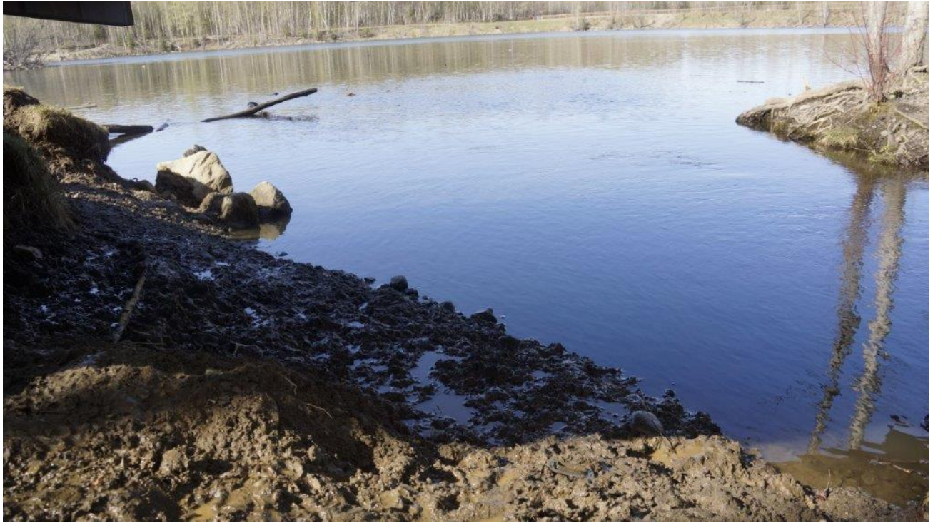
Fig. 17 Bank erosion in 2016 near foot bridge at S. Fork Chester Creek inflow to University Lake, CSF-4
