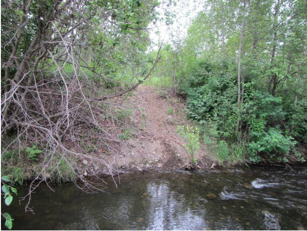
Fig. 15 South bank of S. Fork Chester Creek at University Lake at outflow under Elmore 2013, CSF-4
