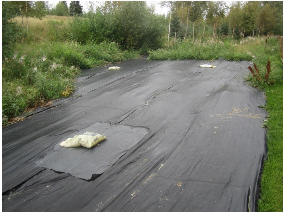
Fig. 19 Area covered with tarping near S. Fork Chester Creek near Begich Middle School in September 2013
