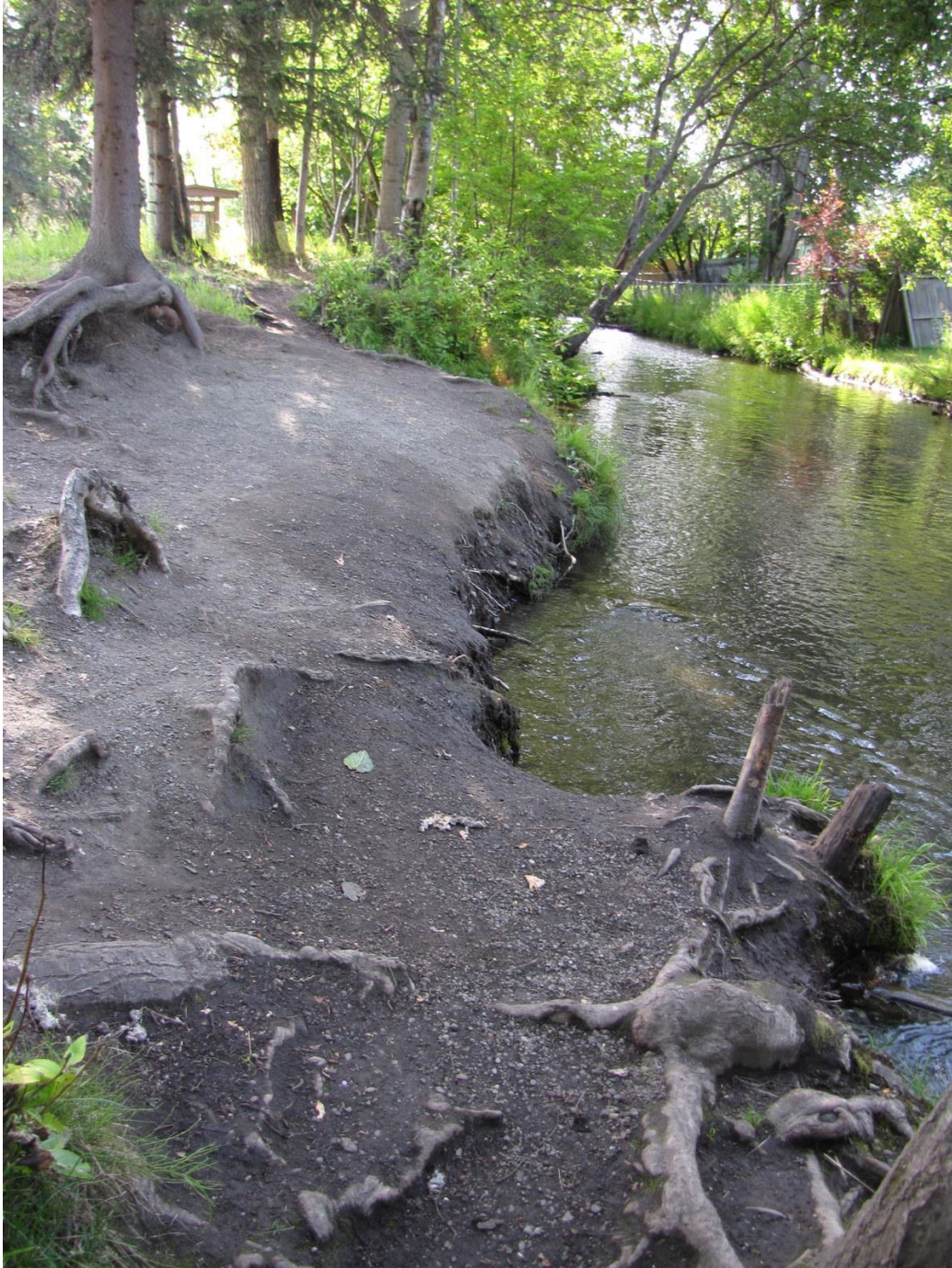
Fig. 3 West bank of Chester Creek showing eroded bank in 2011 (CW-4)
