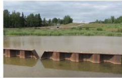
Minnesota Sedimentation basin
